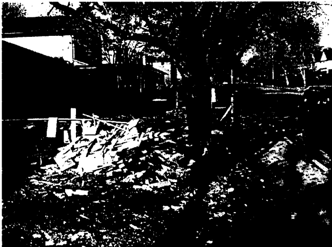
Debris, Compaction and Soil Contamination During Construction
