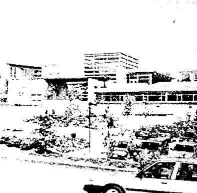
The post-disaster EComm facility is located at 3301 East Pender in Vancouver.
