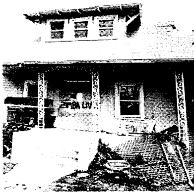
Home damaged by the 6.7 magnitude earthquake that struck Northridge, California on January 17, 1994.
