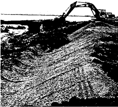
Public Works Crews perform dyke maintenance on the shoreline at Terra Nova.
