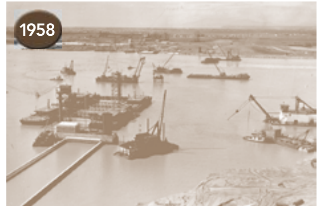
The George Massey Tunnel was the first underwater vehicle tunnel to be built in North America. Six 21,000-foot concrete sections were floated into position, then sunk into a trench, 40 feet below sea level.
