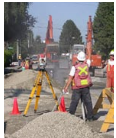
Upgrading transportation and roads improves mobility and safety.
