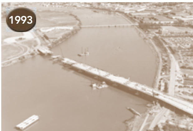
The No. 2 Road Bridge from Lulu Island to Sea Island was built in 1993 to improve access to the Vancouver International Airport and to accommodate the growing commuter traffic between Richmond and Vancouver.
