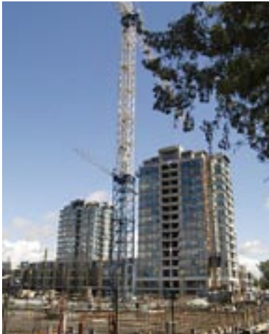
Construction continues to boom in Richmond.
