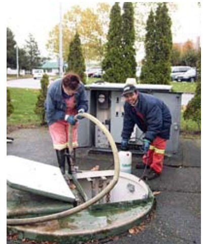
Pump stations are upgraded to enhance operations and safety.
