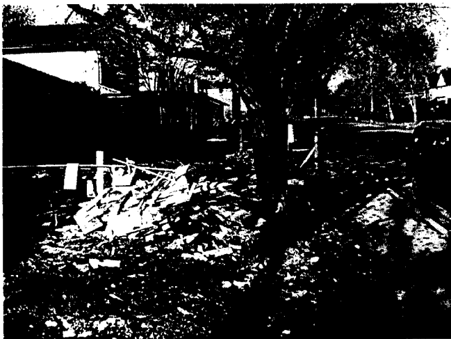
Debris, Compaction and Soil Contamination During Construction
