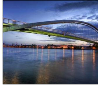
1. No. 2 Road Bridge
