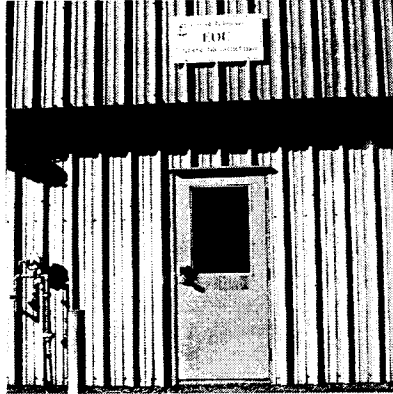
The City's Emergency Operations Centre is located at the City Works Yard on Lynas Lane.
