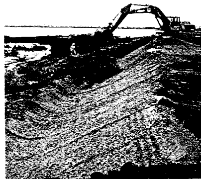
Public Works Crews perform dyke maintenance on the shoreline at Terra Nova.
