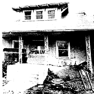
Home damaged by the 6.7 magnitude earthquake that struck Northridge, California on January 17, 1994.
