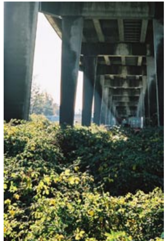
Knight Street bridge
