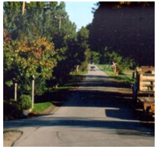
No. 4 Road - South Dyke
