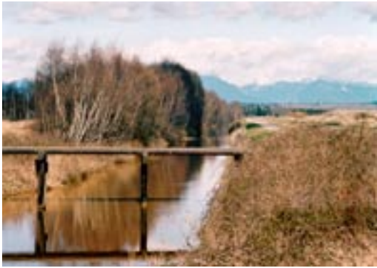
No 7. Road Canal - Fraser Port
