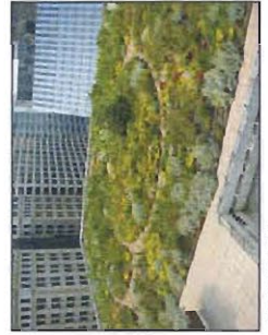
GREEN ROOF DECK
