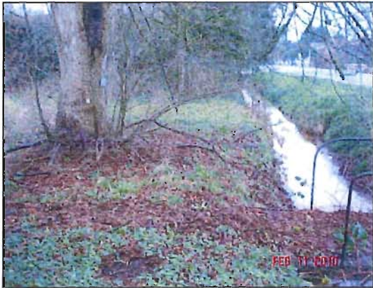
Detail showing the relationship between tree #22 and the open ditch along the edge of Alexandra Road.
