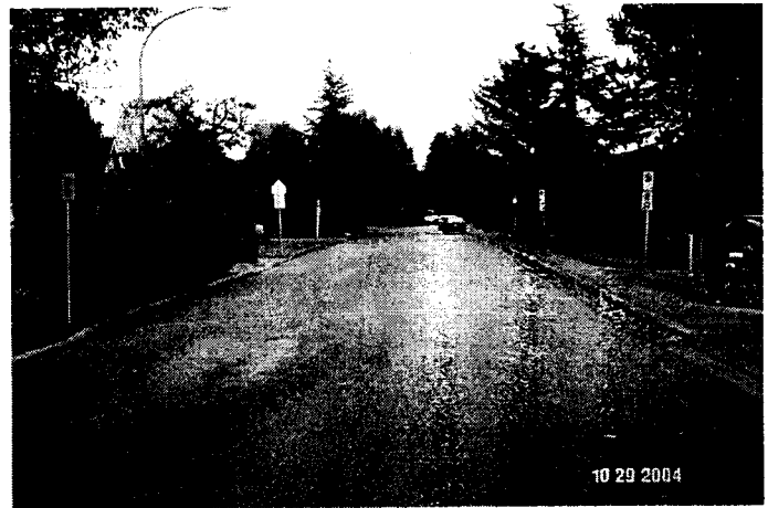
Stopping Prohibition Signage along Frontage of Ferris Elementary School
