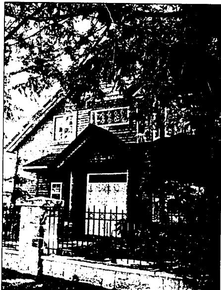
Prominent Building Entrance
