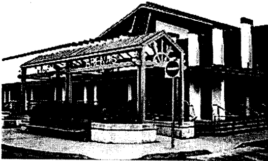
Minoru Arenas at Minoru Gate
