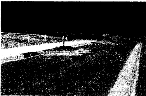
Figure 6.18: Narrowings without Valley Gutter
