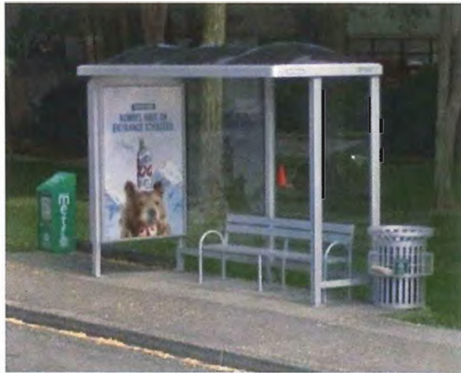
Refurbished Pattison Shelter
