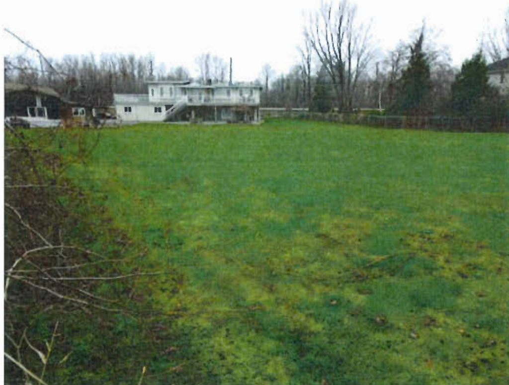
Figure 8. View of the home towards the north, with the backyard. The owners described regular flooding of the backyard (see also Appendix B)
