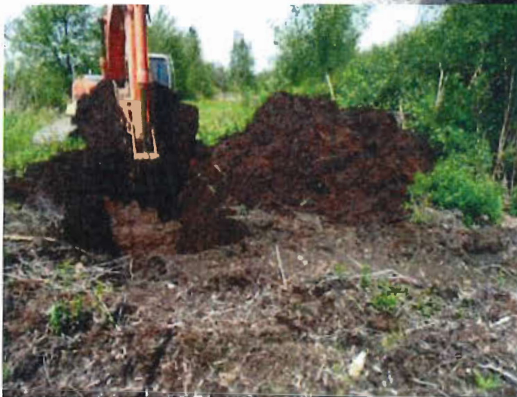
Figure 11. The clay layer was approximately 240 cm below the surface of the peat.
