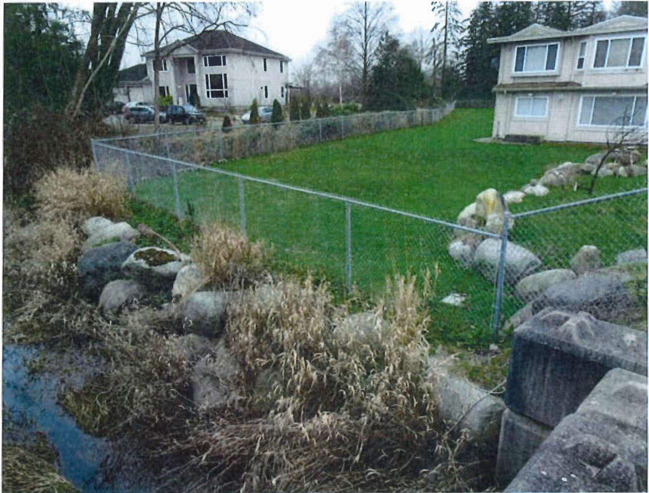
Figure 7. View of front of property (northeast corner) from the road. Owners indicated regular flooding of the front yard (see photos in Appendix B).
