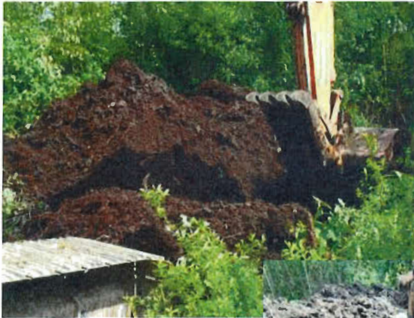
Figure 17. Excavating soil pit # 1 at 21700
