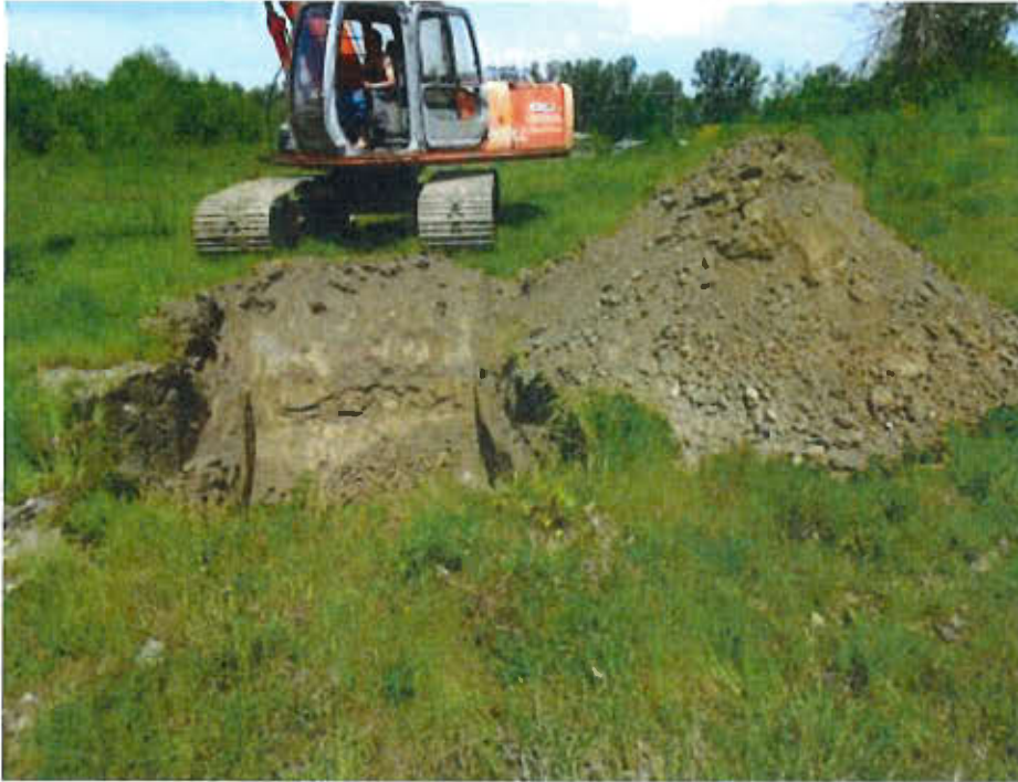
Figure 20. Inspection of the imported soil in Hole # 3 did not reveal any contamination.
