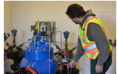
Maintaining the PRV station
