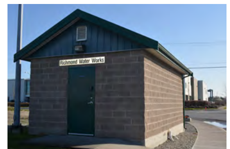
Exterior of the Blundell PRV station
