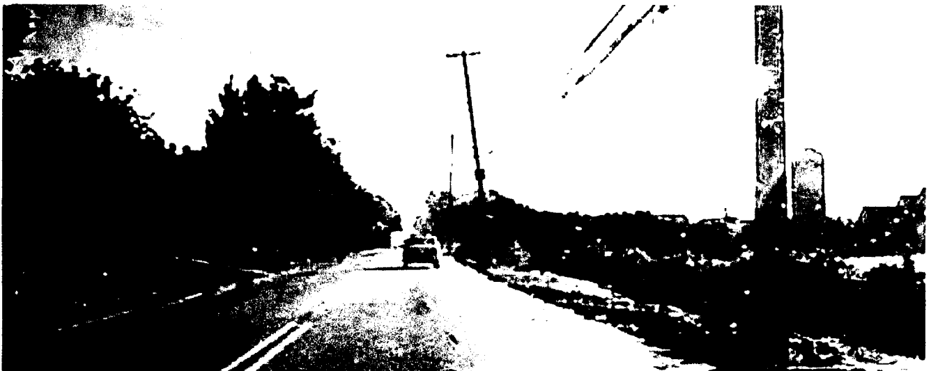
Westminster Highway (No. 6 Road to No. 7 Road looking east) – A new 3.0 metre separated bicycle path for two-way cycling traffic will be introduced along the filled ditch area on the south-shoulder of Westminster Highway behind existing hydro poles.
